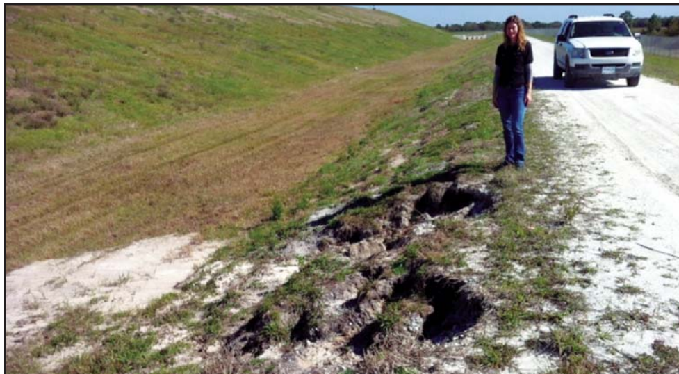
Figure 5. Interior Slope Washout
